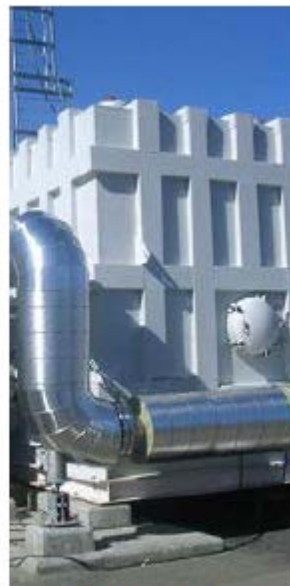
1400 kW MCFC (Courtesy FuelCell Energy, Inc.)
